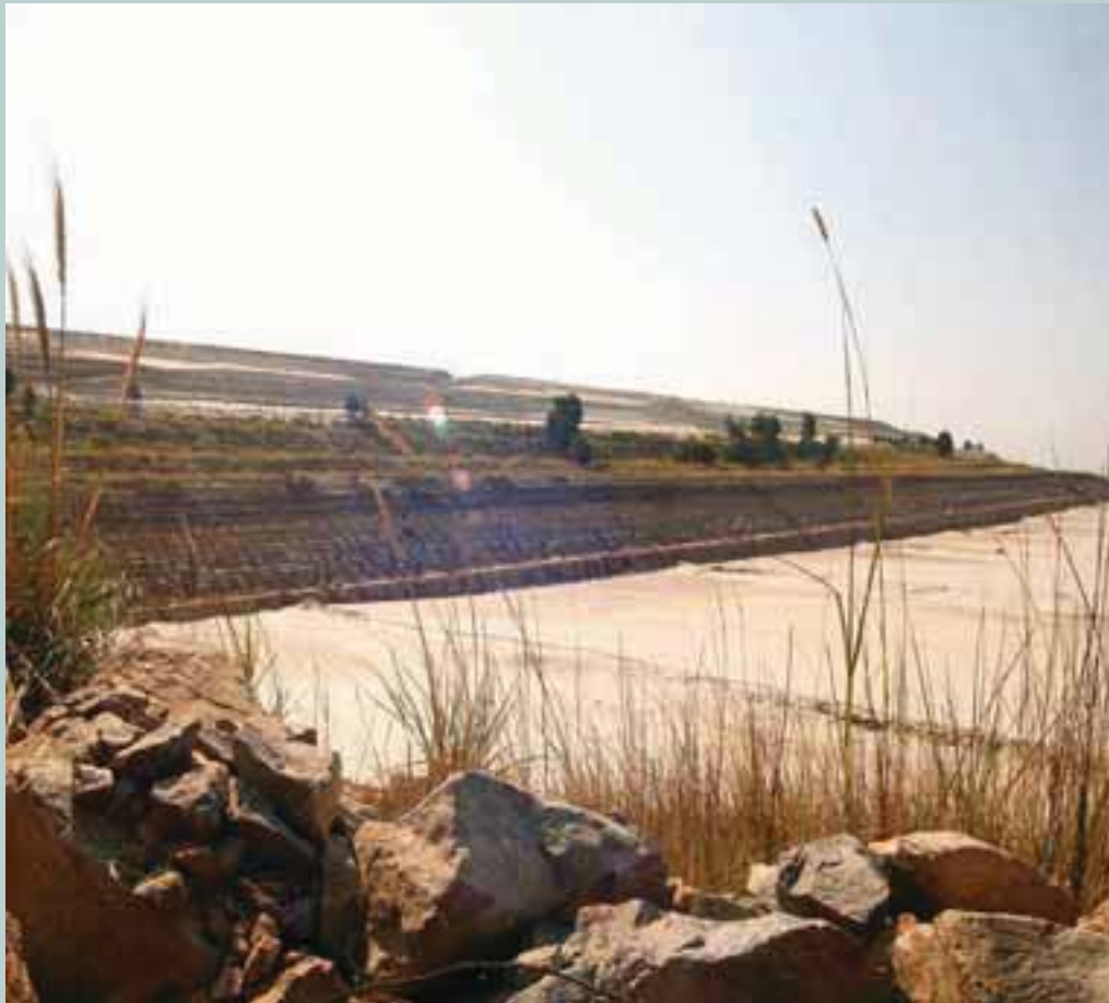
Tailings dam, Randfontein, South Africa
