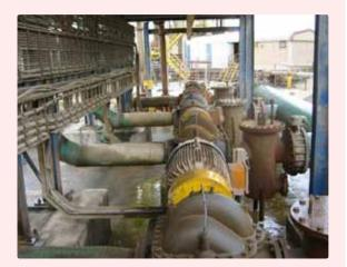
Two energy efficiency projects – Kusasalethu water turbines and Evander 8 shaft solar water heating – were successfully implemented, resulting in a load reduction of 1.84MW and energy savings of 1 323MWh per month. Kusasalethu is also commissioning two more water turbines that will contribute 3MW load reduction and 31 536MWh energy savings per annum.
