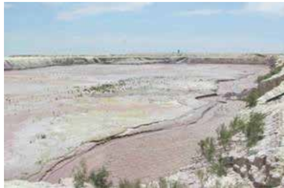
The Brand A tailings facility is currently being reclaimed. This involves resludging and pumping material to the metallurgical plant for processing. Historically, tailings facilities were not considered environmentally friendly areas; our aim is to reclaim down to red soil and leave an environmentally friendly footprint for redevelopment
