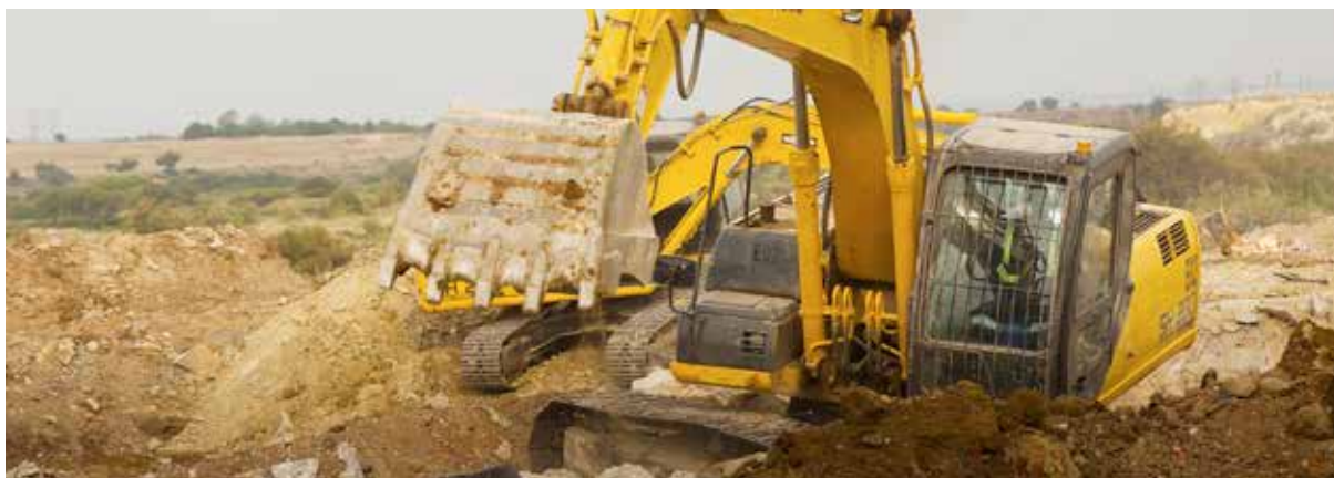
Work in progress at a rehabilitation site in Welkom
