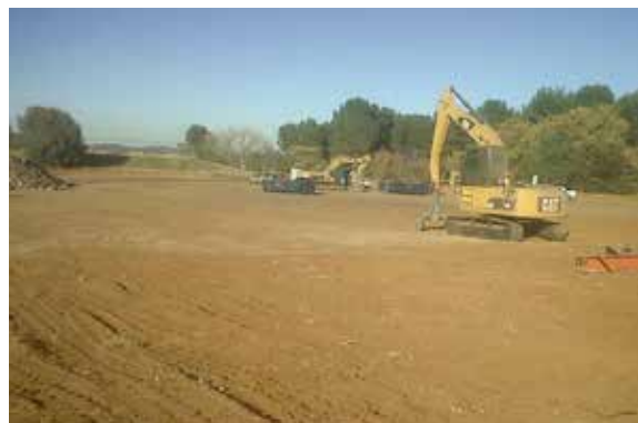
The first step in rehabilitating land is to demolish surface infrastructure to restore the land to a predetermined use
