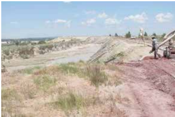
The Brand A tailings facility is currently being reclaimed. This involves resludging and pumping material to the metallurgical plant for processing. Historically, tailings facilities were not considered environmentally friendly areas; our aim is to reclaim down to red soil and leave an environmentally friendly footprint for redevelopment
