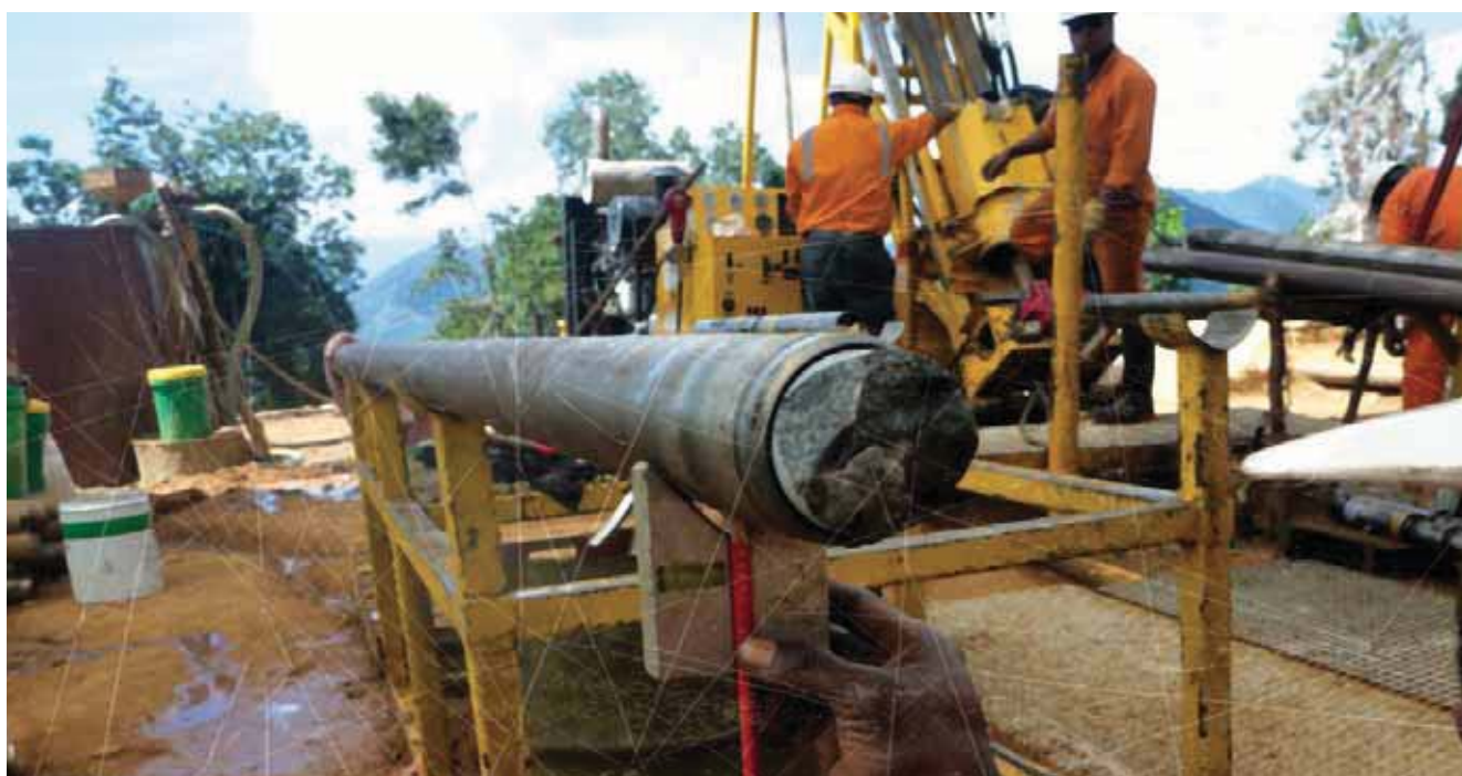
Kurunga prospect drilling operations
