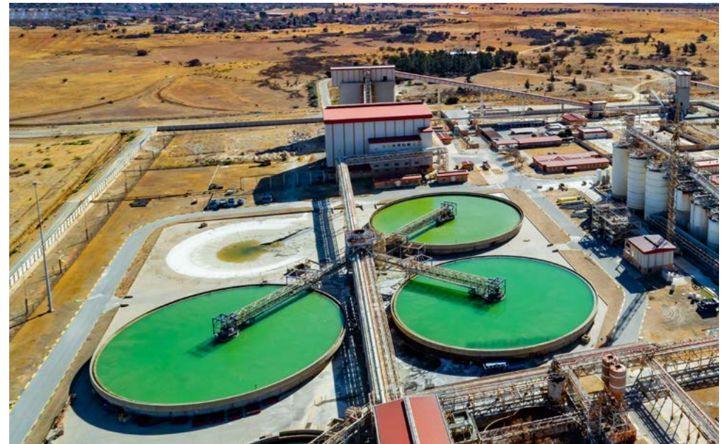
■ Central Plant, Welkom
