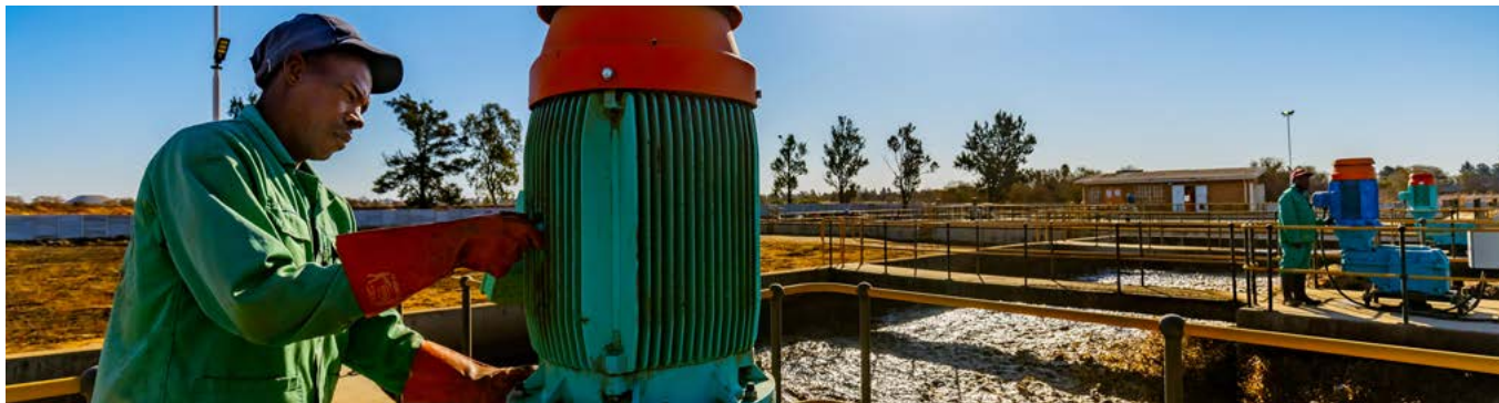
■ Water management at Oberholzer Wastewater Treatment Plant
