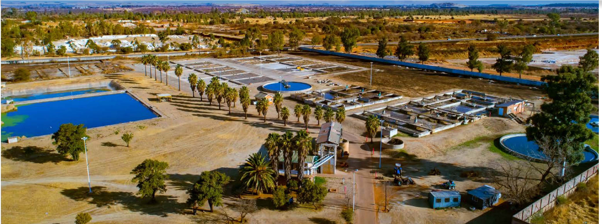
■ Stilfontein wastewater treatment plant
