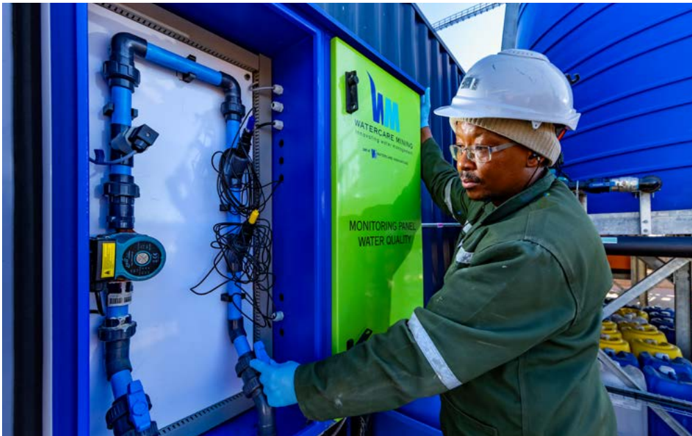
■ Target water treatment plant
