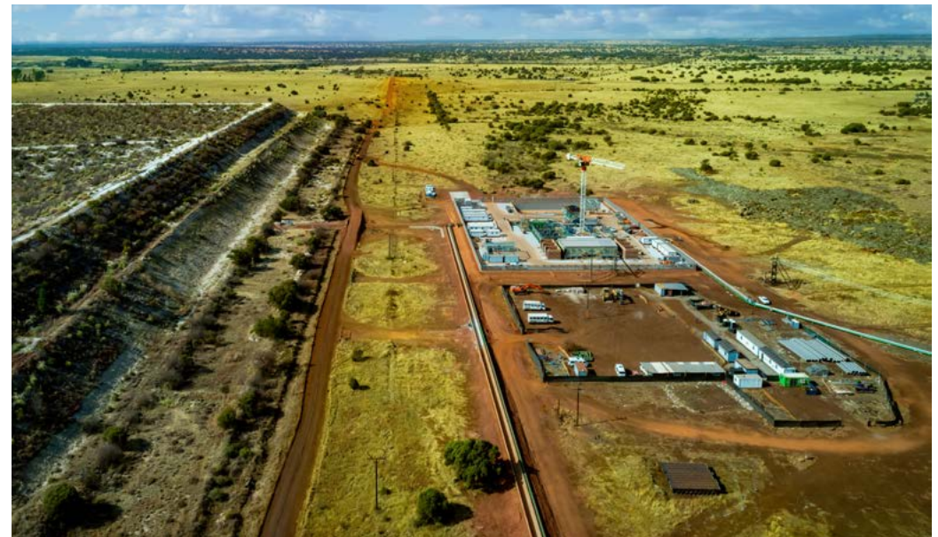
■ Orkney Mine Waste Solution pump station project
