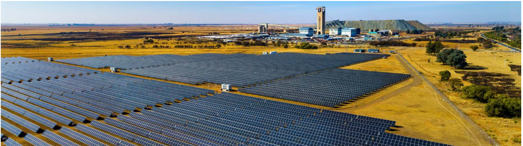
■ Tshepong North PV solar renewable energy project
