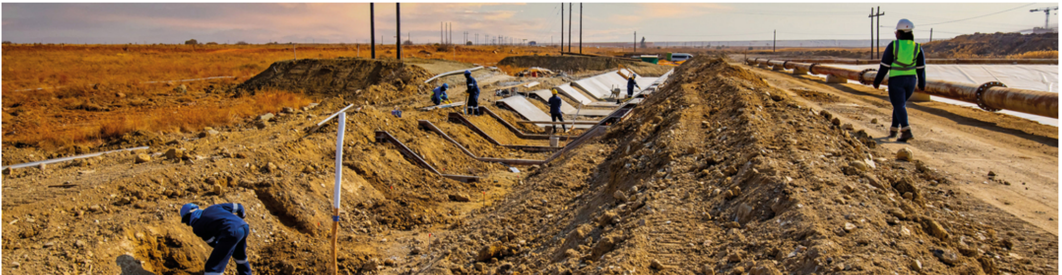
■ Kareerand extension, Mine Waste Solutions
