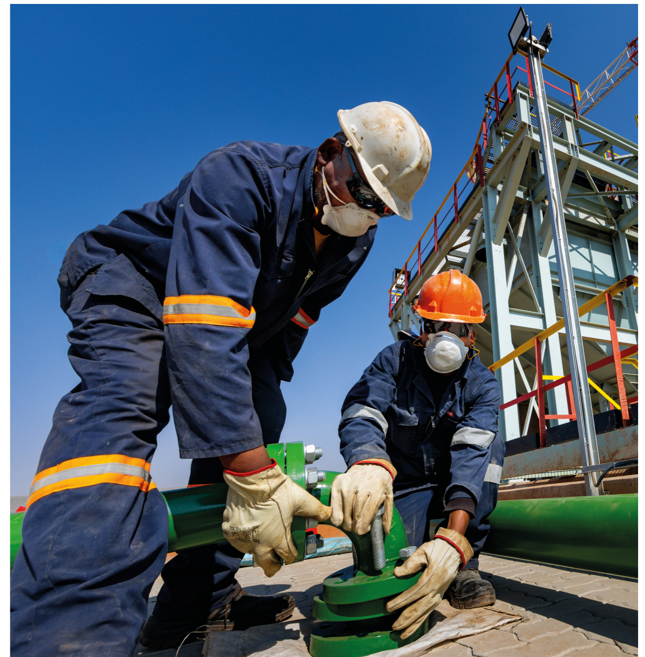
■ Mine Waste Solutions pump station project
