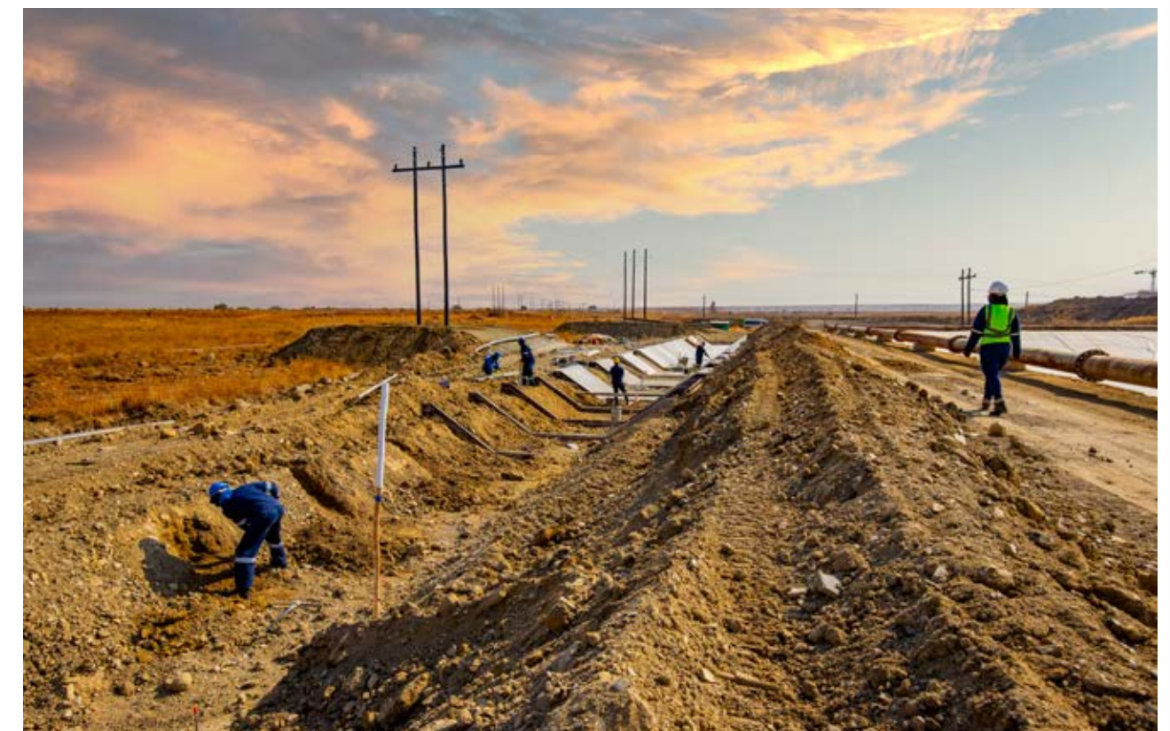
■ Kareerand extension, Mine Waste Solutions
