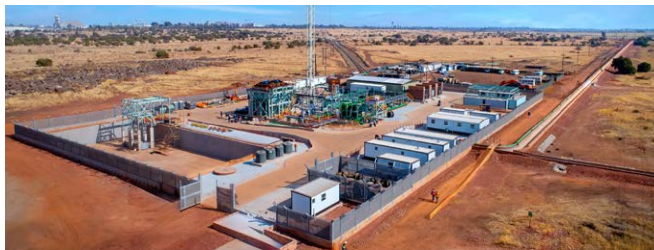
Orkney MWS 4 and 5 pump station project.
