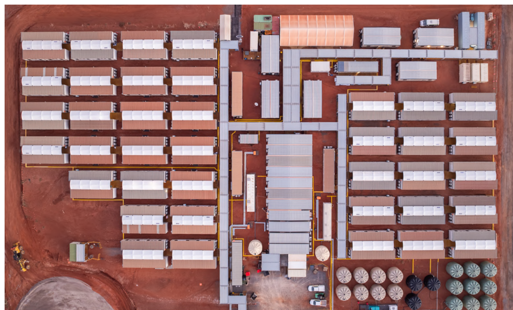
Bird's-eye view of Eva Copper Project accommodation
