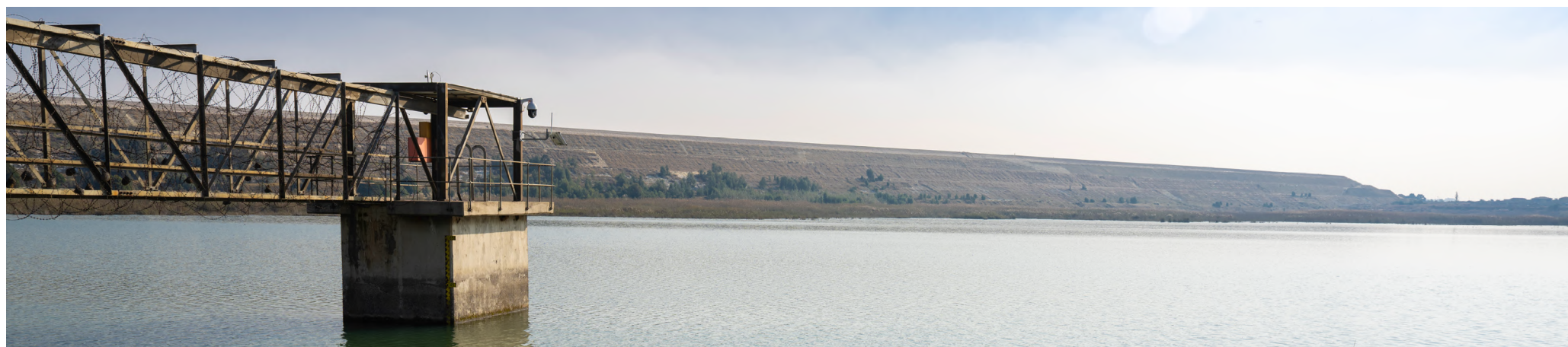
Return water dam, Doornkop, Gauteng, South Africa
