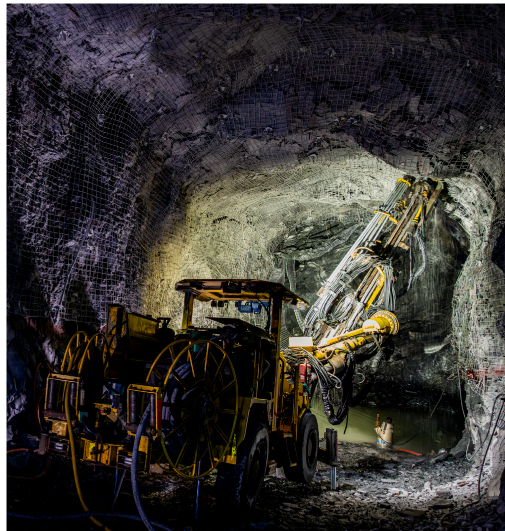
Rock bolting, Moab Khotso, North West, South Africa
