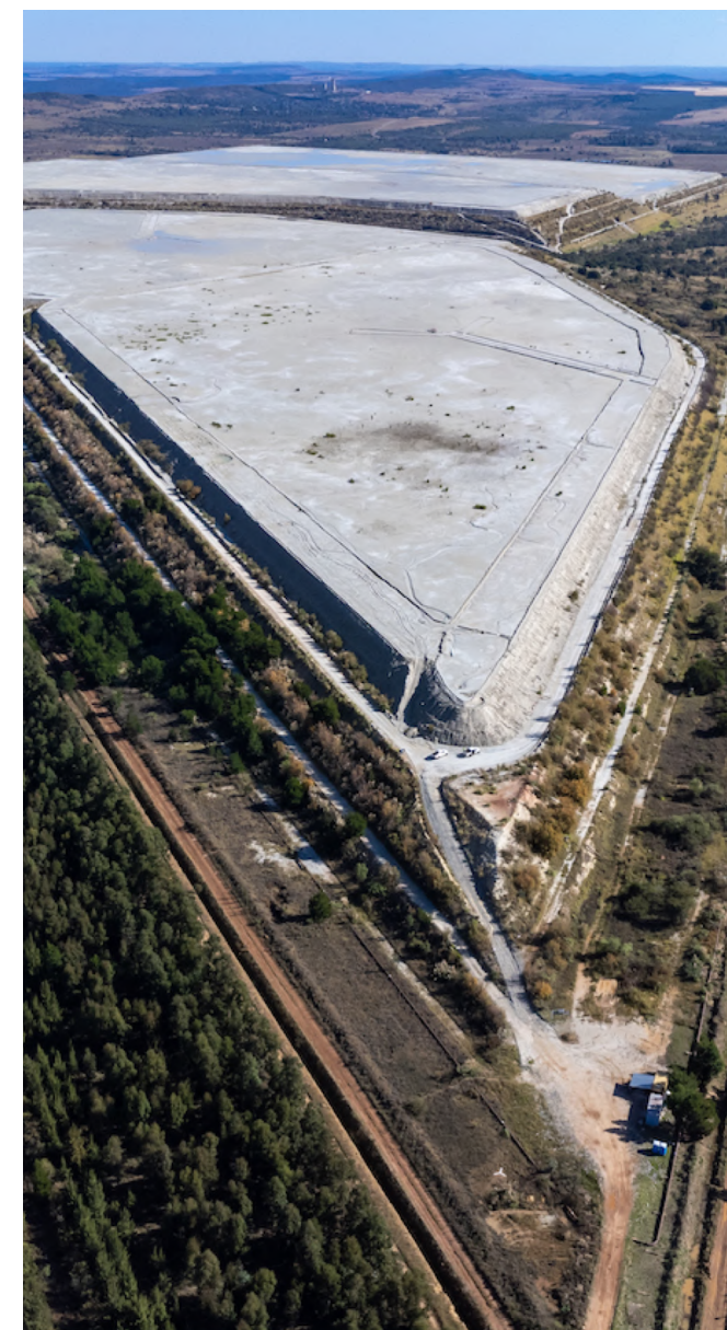
Tailings storage facility, Savuka, Gauteng, South Africa
