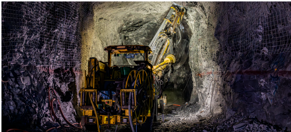
Rock bolting, Moab Khotsong, North West, South Africa
